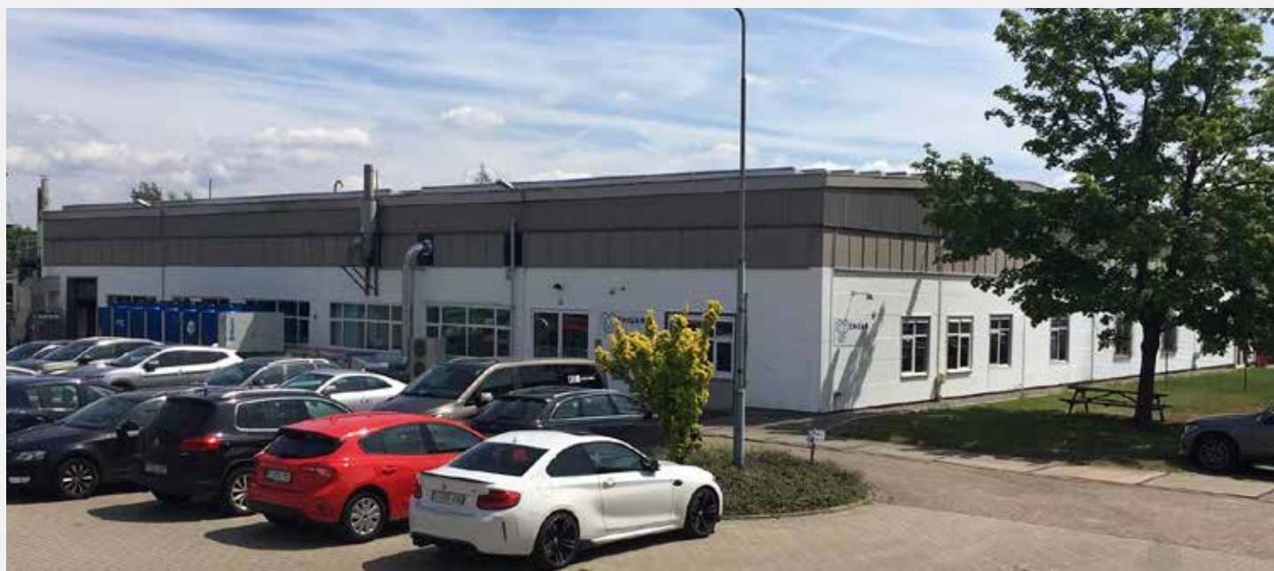
SOITEC BELGIUM N.V HASSELT, BELGIUM
