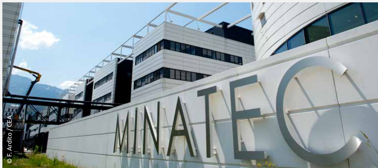
SUBSTRATE INNOVATION CENTER - FRANCE
